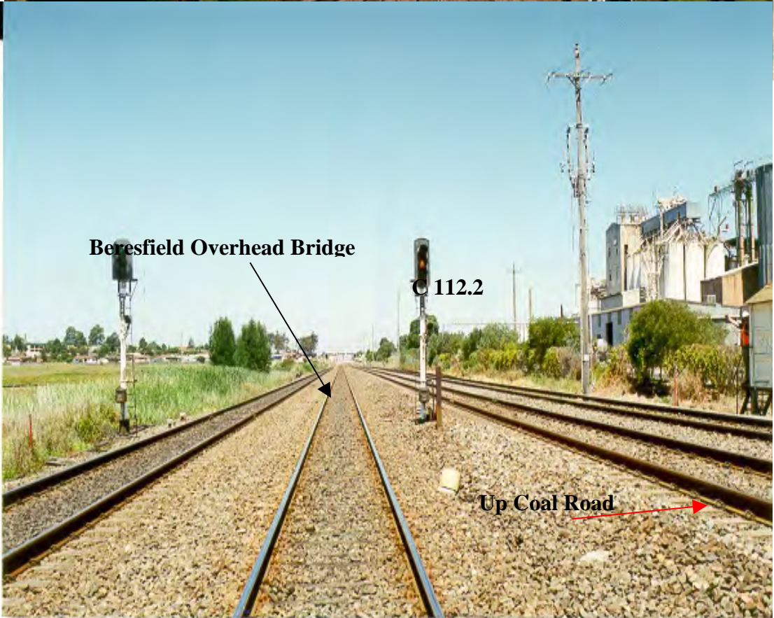
Figures 11 and 12 showing signals C113.0 and C112.2.
