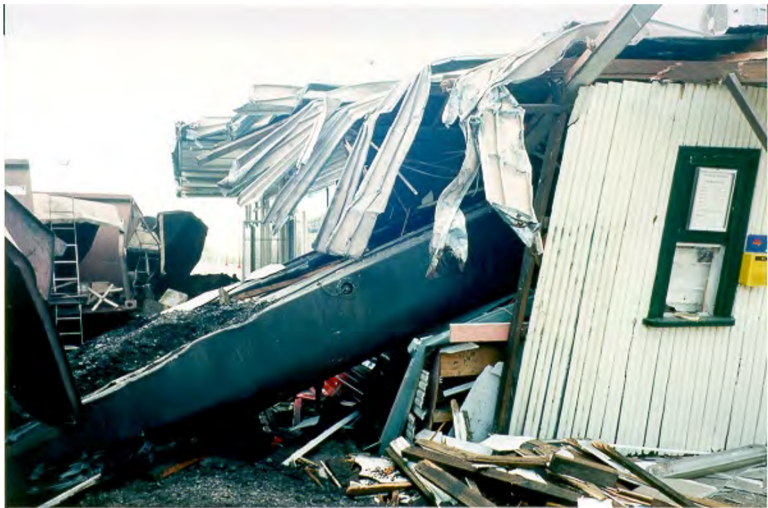
Figures 8 and 9. Both coal roads and main northern lines were completely blocked. Extensive damage to the Beresfield station booking office and platform is evident
