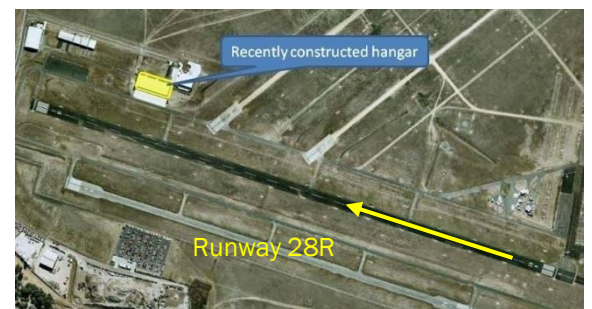
Figure 1. Runway 28R, showing the recently-constructed hangar
