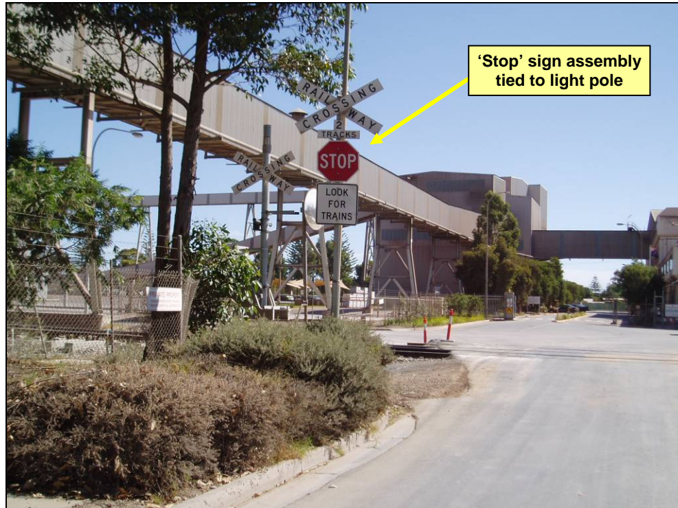
Figure 10: Stop sign assembly on the day of the collision
