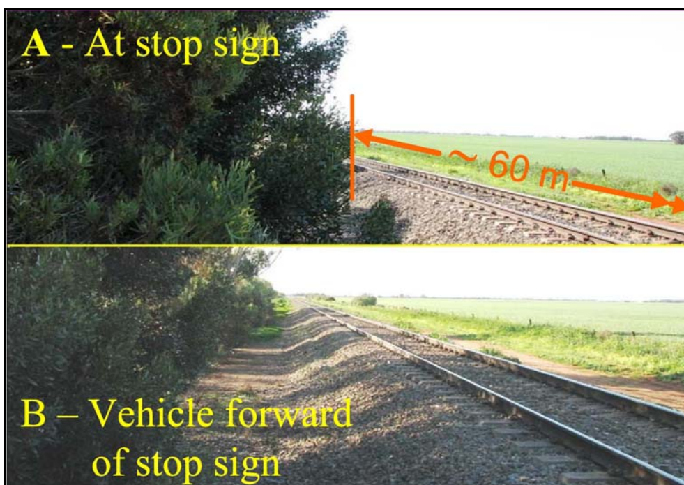
Figure 6: Sighting distance looking north at the Murrow Farm level crossing
