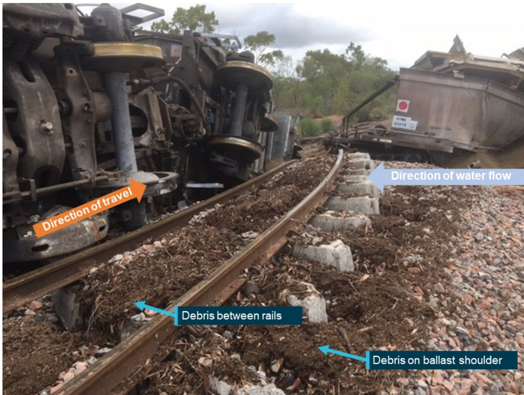
Figure 10: Evidence of debris on ballast shoulder and between rails
