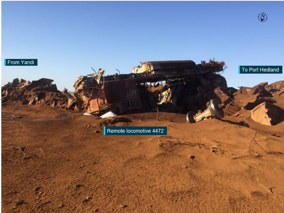
Wreckage of remote locomotive 4427 and ore cars from rakes A and B viewed in a south-westerly direction at Turner South. Source: BHP, annotated by the ATSB
