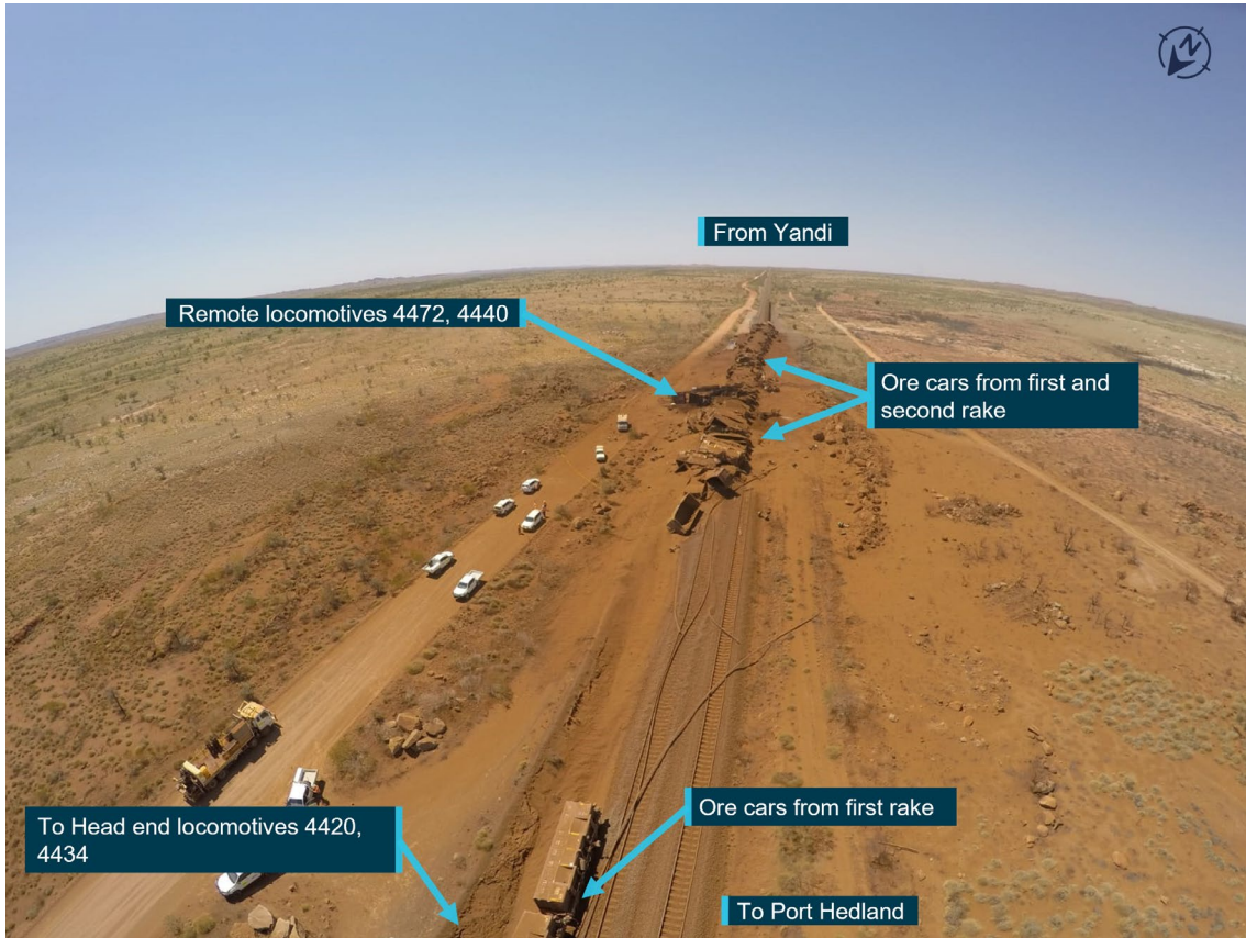
Aerial image viewed in a southerly direction of train wreckage and track damage at Turner South. The lead locomotives 4420 and 4434 remained on track and were coupled with one ore car that had derailed (out of frame in the foreground). Source: BHP, annotated by the ATSB
