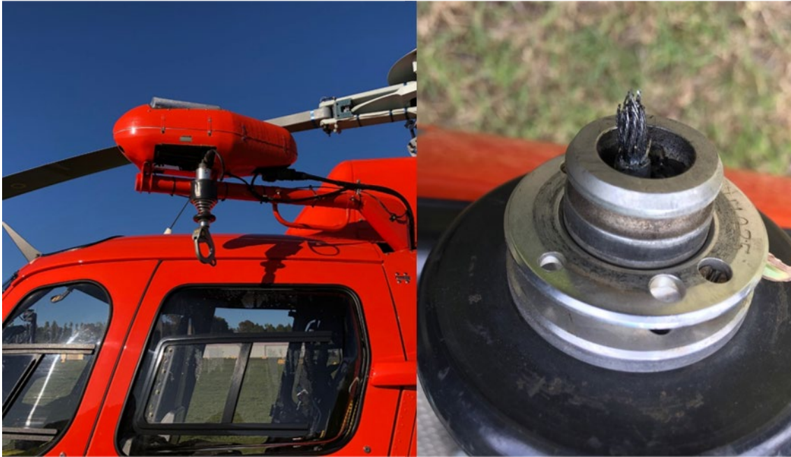
The fractured cable was found protruding from the swivel hook assembly. Source: National Parks and Wildlife Service
