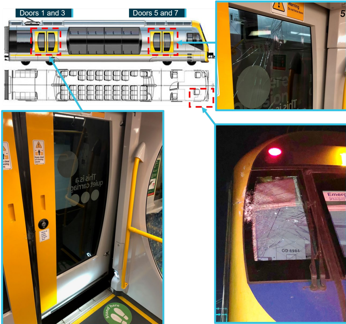
The diagram and photos show the location of the damage on carriage 6984. The bottom of passenger doors 1 and 3 were pulled outwards by the air filter hatch.
