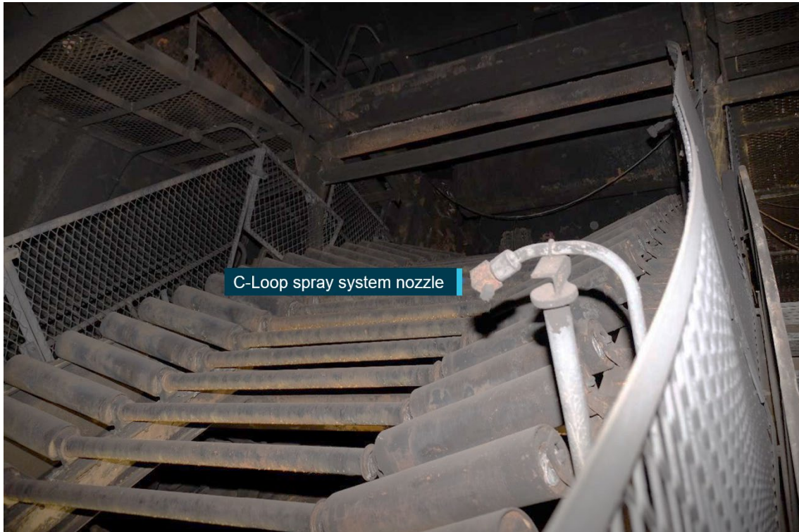
Figure 14: C-Loop spray system nozzle
