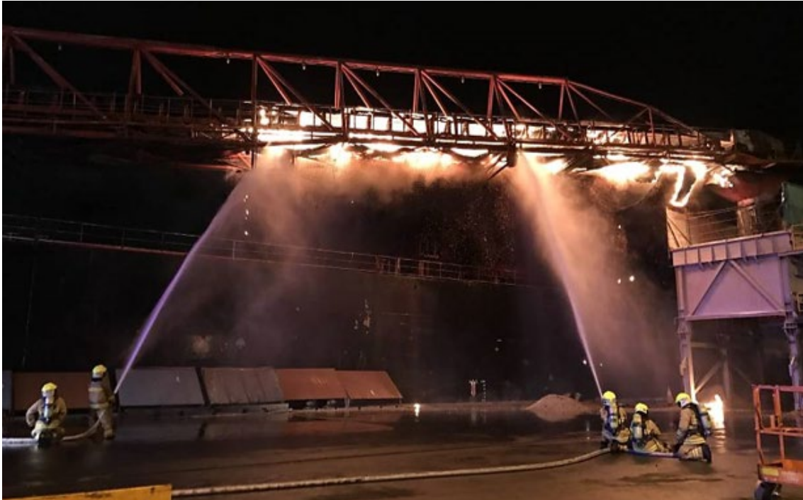
Figure 5: Boom conveyor on fire
