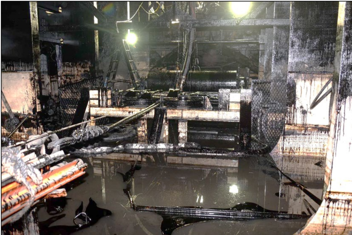
Figure 19: Bottom of C-Loop space, looking aft
