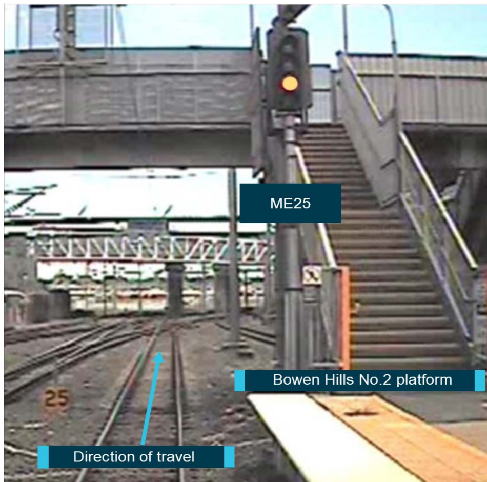
Figure 1: Signal ME25 showing a yellow aspect as TP43 arrived at Bowen Hills
