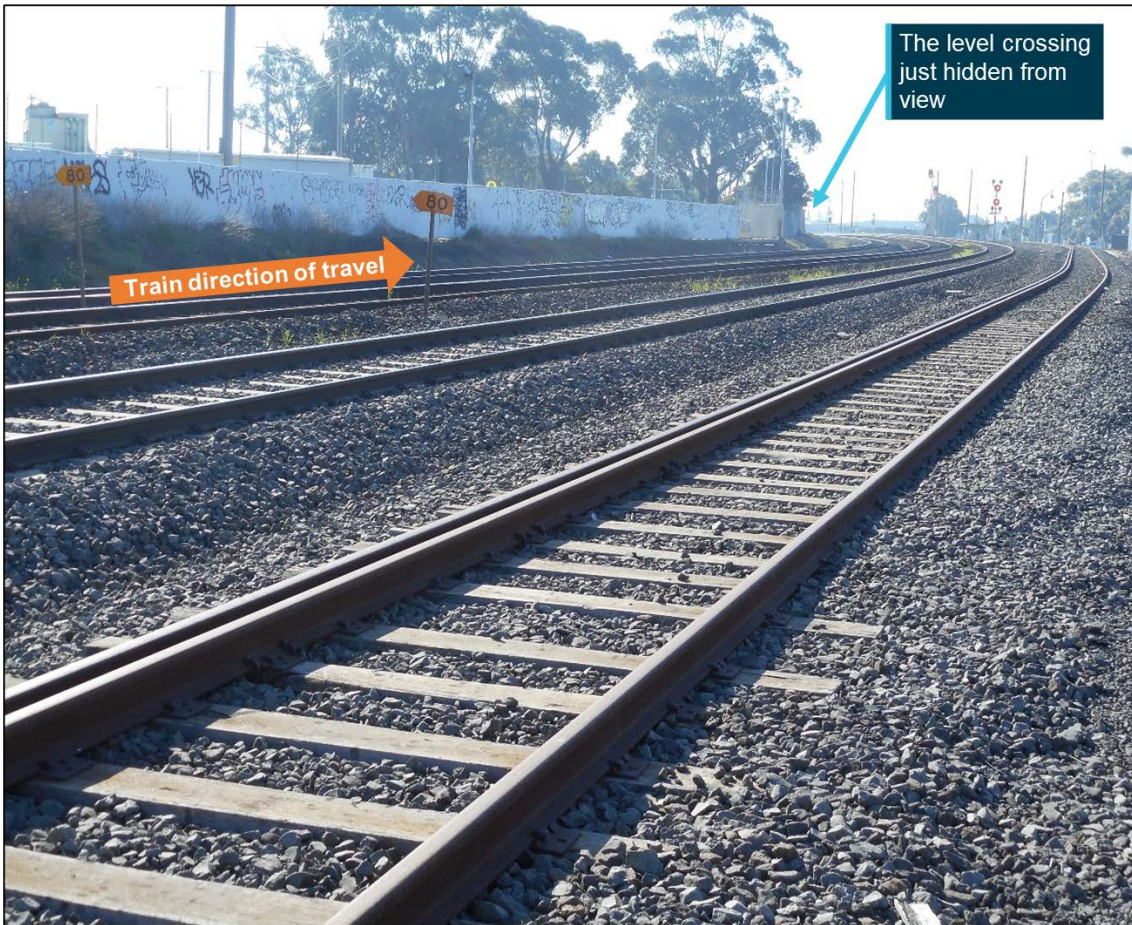
Figure 8: The rail approach to the Station Street level crossing
