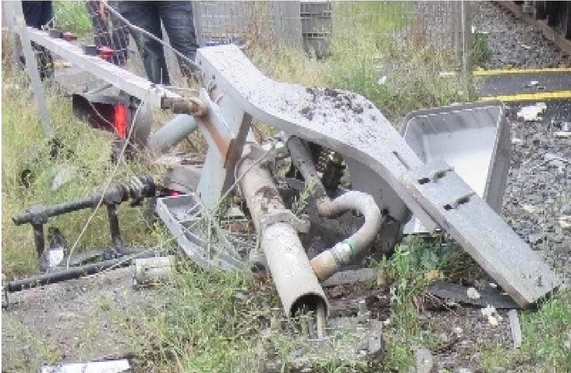
Figure 5: Damaged flashing signal and boom barrier assembly
