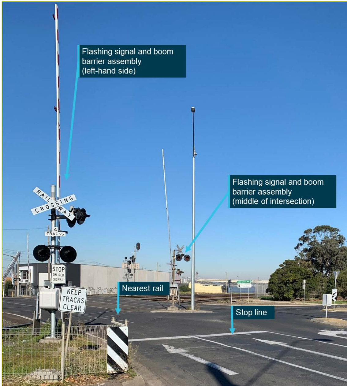
Figure 7: Road approach to level crossing including signage and protection equipment flashing light and boom barrier assembly
