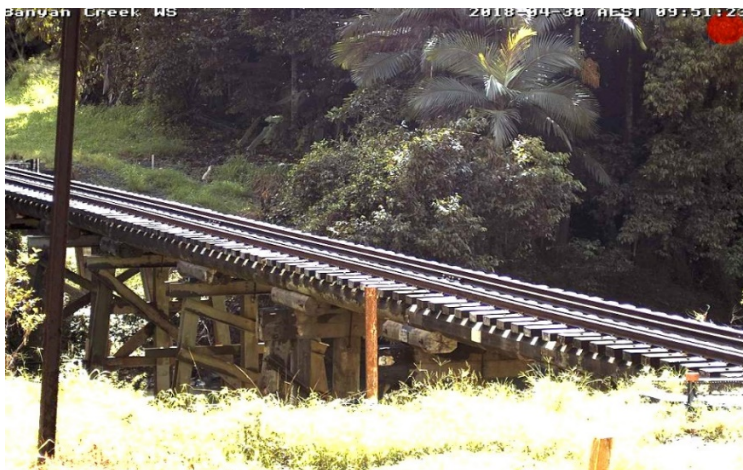
Figure 4: Little Banyan Creek rail bridge
