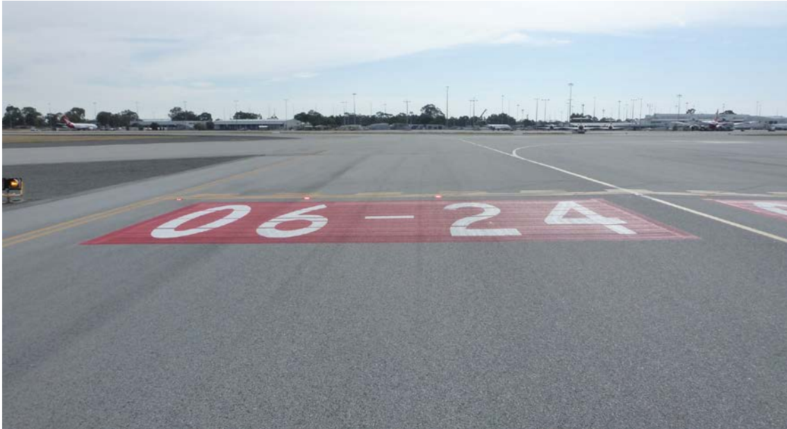
Figure 8: Runway identifier (red and white markings) and stop bar (red lights) installed on taxiway J2
