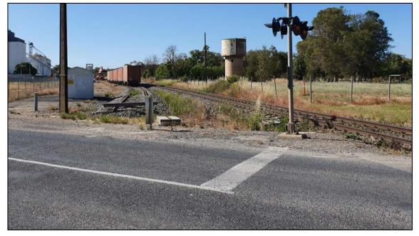
Runaway wagons stopped about 40 m from the baulk. The image illustrates how wagons that might roll to the end of the track may encroach on the road and level crossing. Source: ATSB
