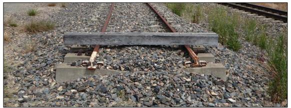
Restraining device installed at Bordertown. A rectangular piece of hardwood timber of approximately 300 by 200 mm, bolted to the track, known as a baulk. Source: ATSB
