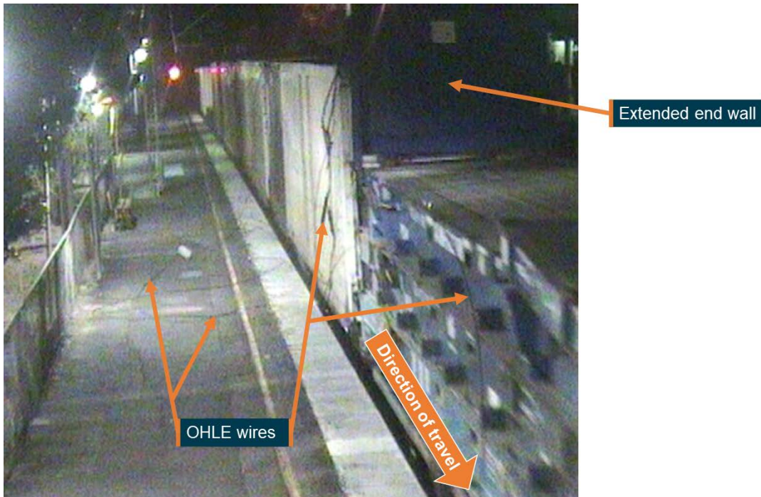
Figure 4: CCTV footage at Cooroy station showing the flat racks with the extended end wall and OHLE wires that had been brought down
