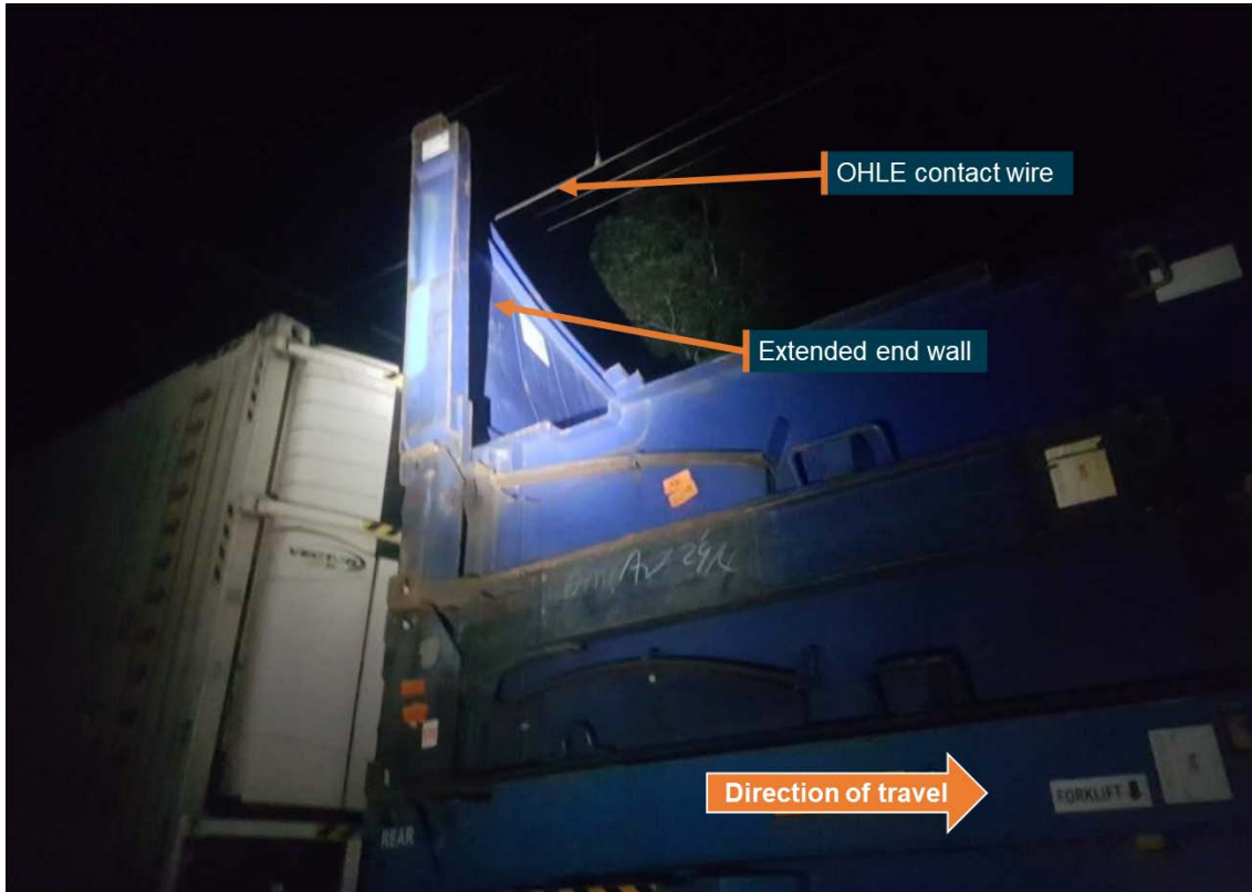
Figure 5: Flat rack end wall in the extended position in close proximity to the OHLE
