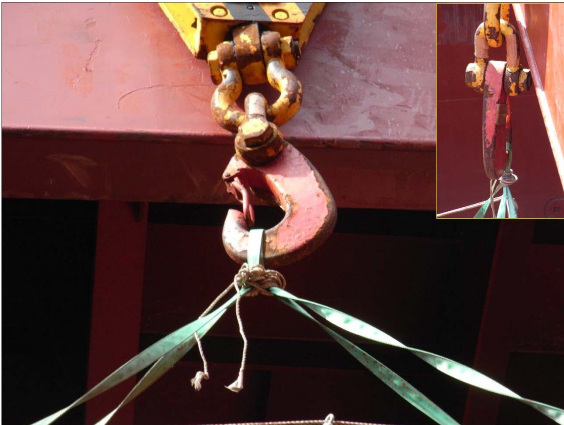
Figure 10: Crane hook and shackle in approximate position as at time of incident. Inset shows the view from the side with protruding hook shackle pin.
