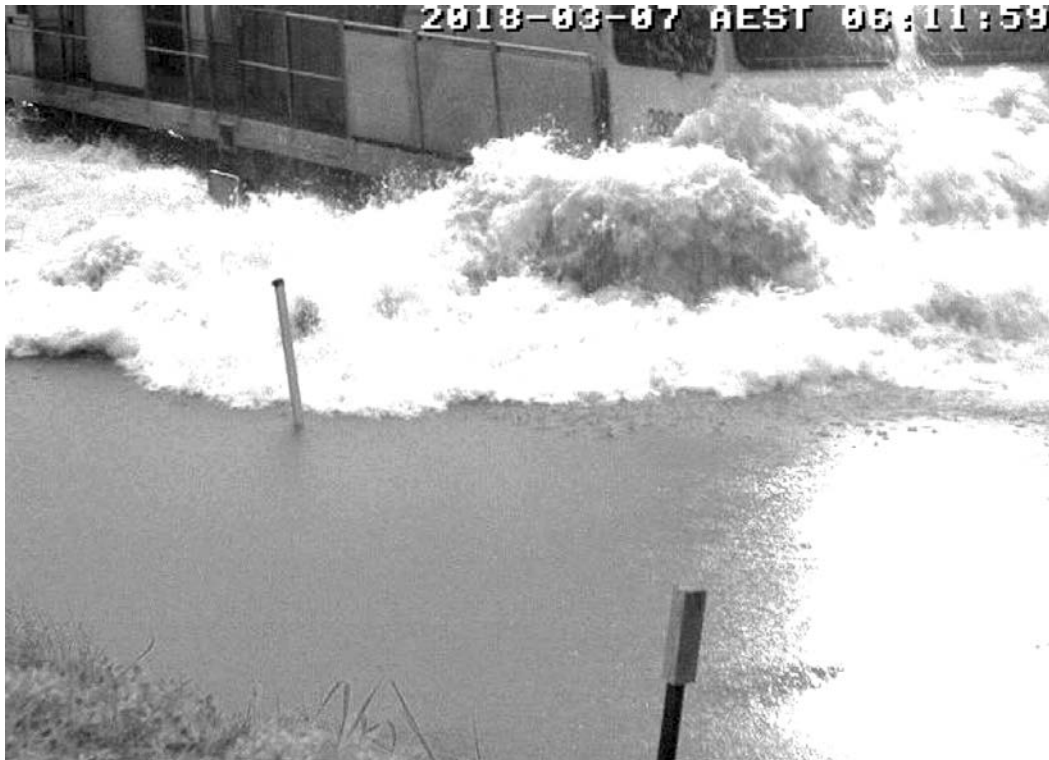
Figure 4: Train 6792's locomotive passing over the flooded Little Banyan Creek rail bridge
