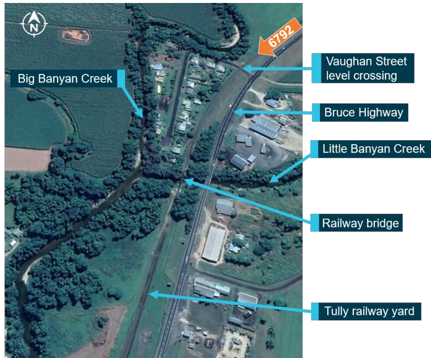
Figure 3: Train 6792's route on approach to the Little Banyan Creek rail bridge
