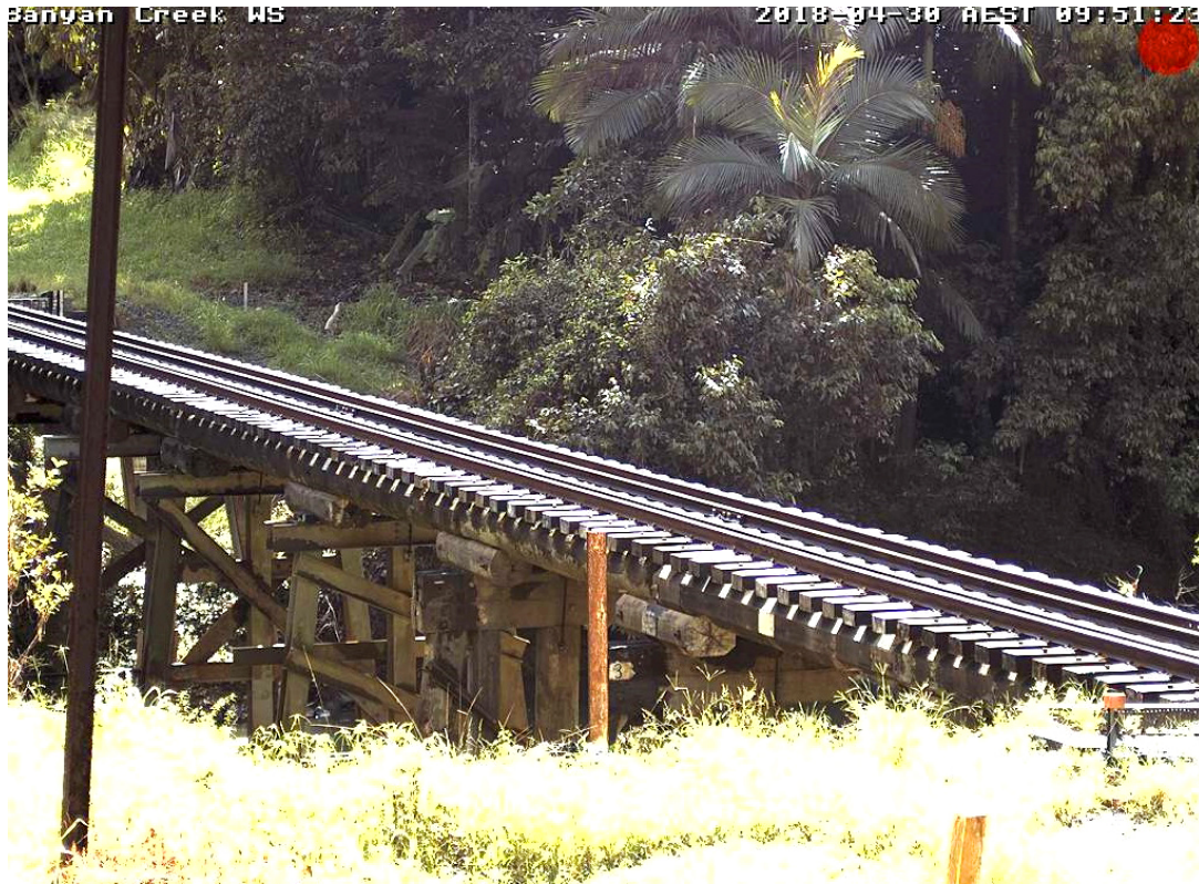
Figure 6: Little Banyan Creek rail bridge
