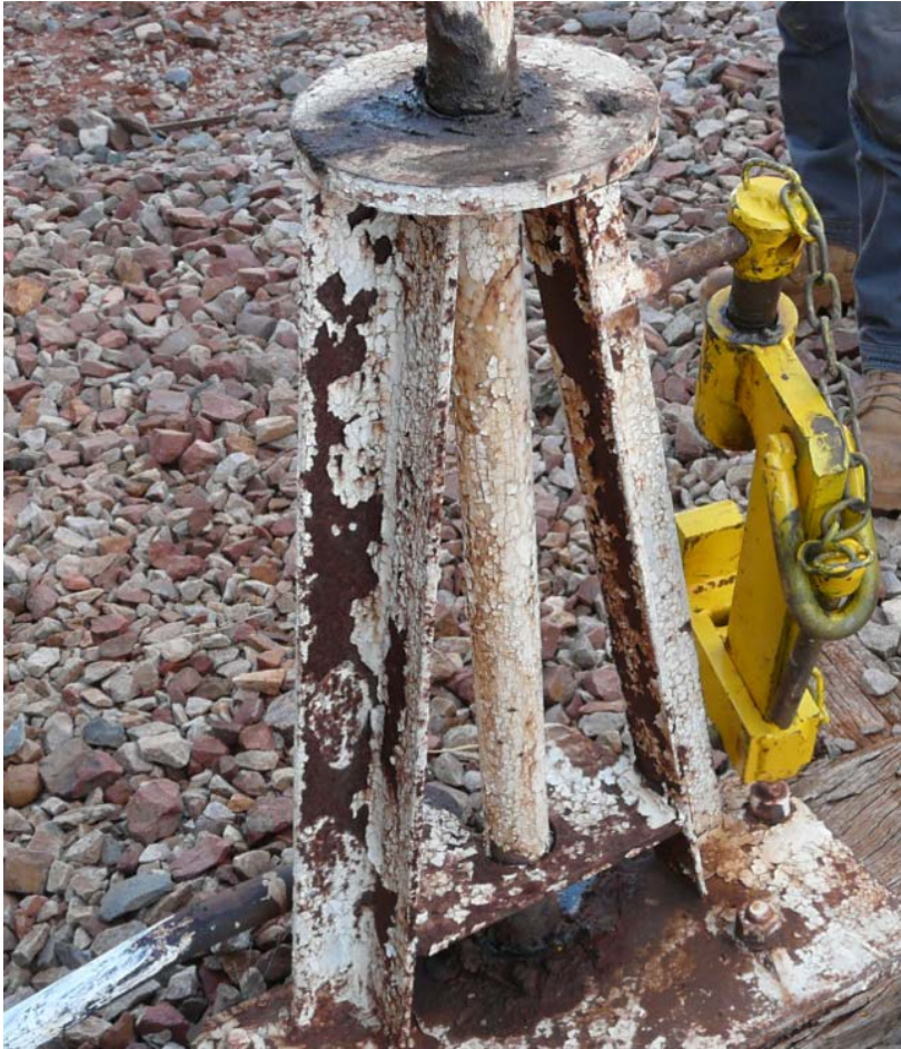
Figure 7: ARTC example of correct storage arrangement for a point clamp on a point indicator stand.
