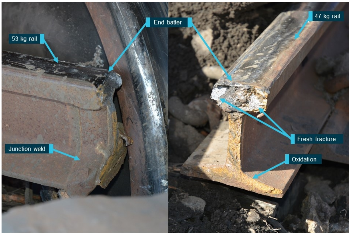
Figure 11: Broken Up rail
