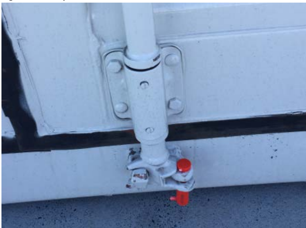
Figure 8: Security seal on the end door of the container
