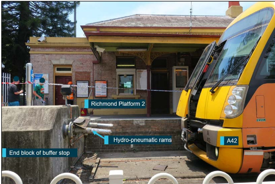
This figure shows the post-collision damage to the buffer stop on Platform 2 and the front of A42. Source: ATSB
