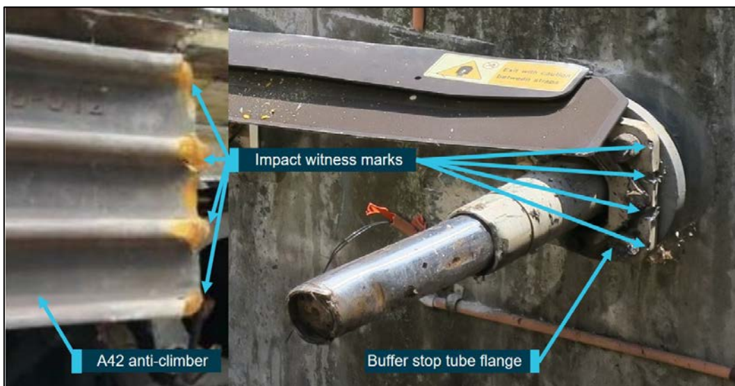
This figure shows the damage to the buffer stop tube flange (Right side) following contact with A42's RHS anti-climber (Left side) and the corresponding damage to the RHS anti-climber edge. Source: ATSB
