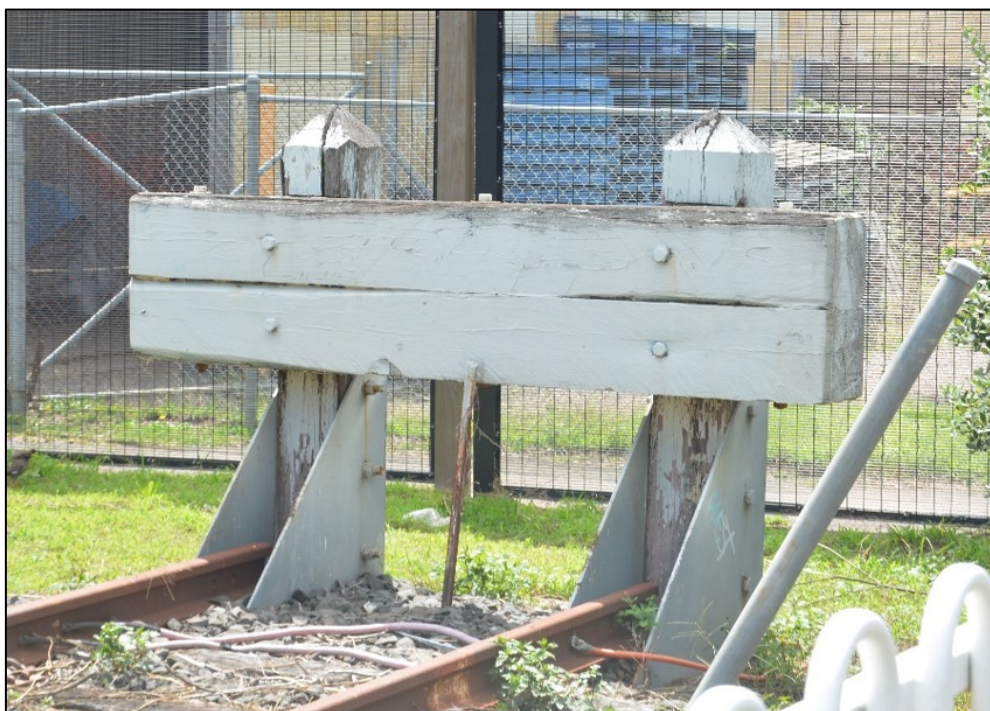
Figure 21: Fixed buffer stop at Carlingford station
