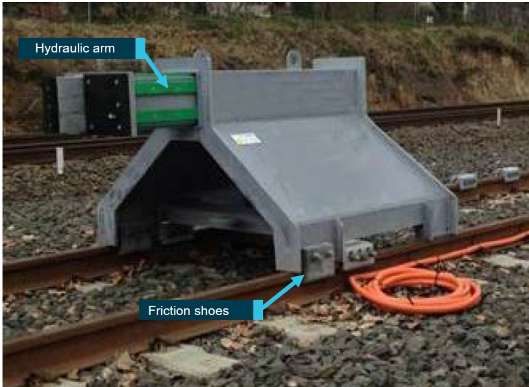
This figure shows an energy-absorbing combination of hydraulic and friction buffer stop. It has friction shoes designed to stop or slow the train upon impact. The front of the buffer stop has a hydraulic arm with a rubber face coupling arrangement. Source: TfNSW with annotations by ATSB
