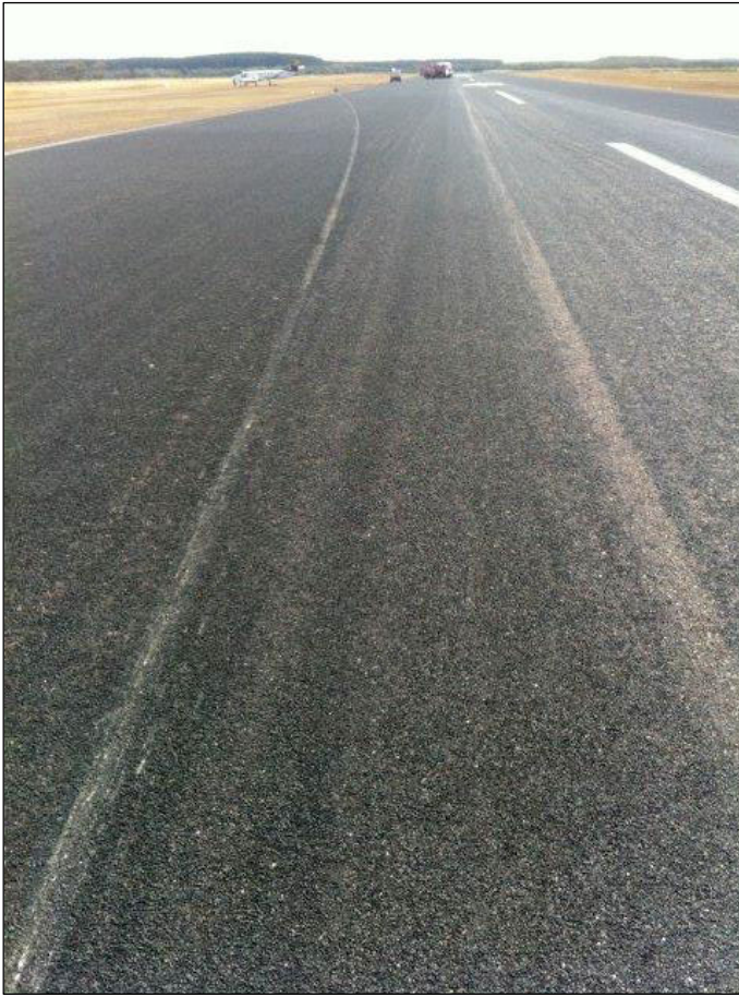
Figure 2: Damage to runway as a result of contact with the left main landing gear following failure
