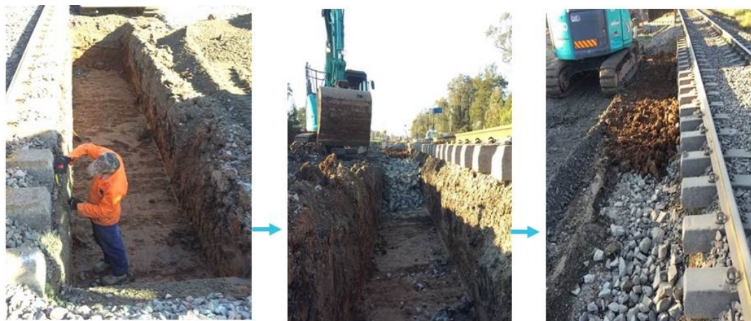
Figure 12: Shear key construction at Denman
