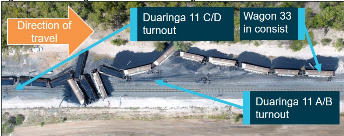
Figure 2: Derailed wagons 33 to 46 on the Duaringa to Aroona down line
