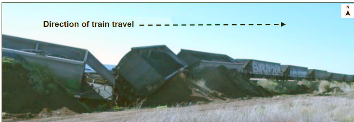
Figure 3: Derailed coal wagons of train 9869
