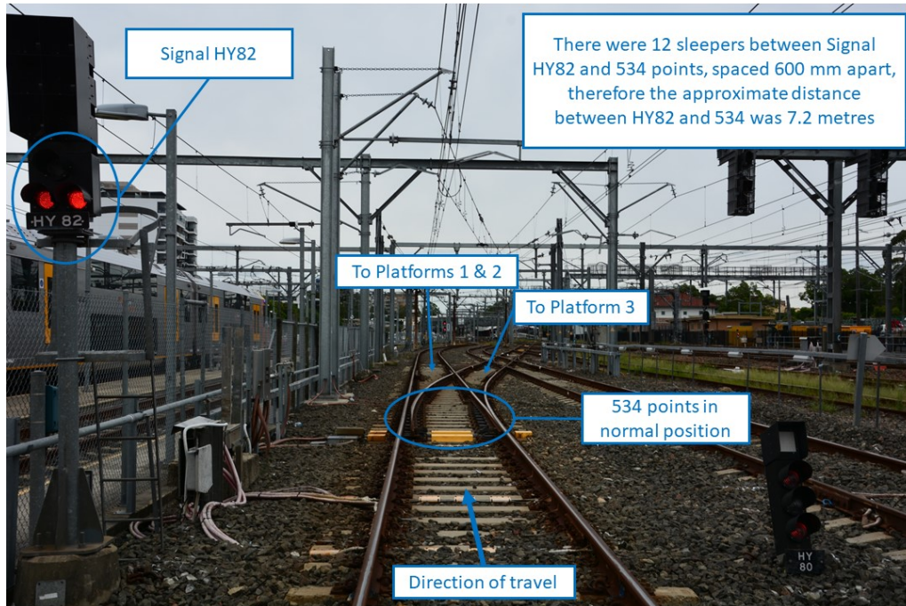
Figure 4: Signal HY82 and 534 points. 534 points set for movement straight ahead (normal position)
