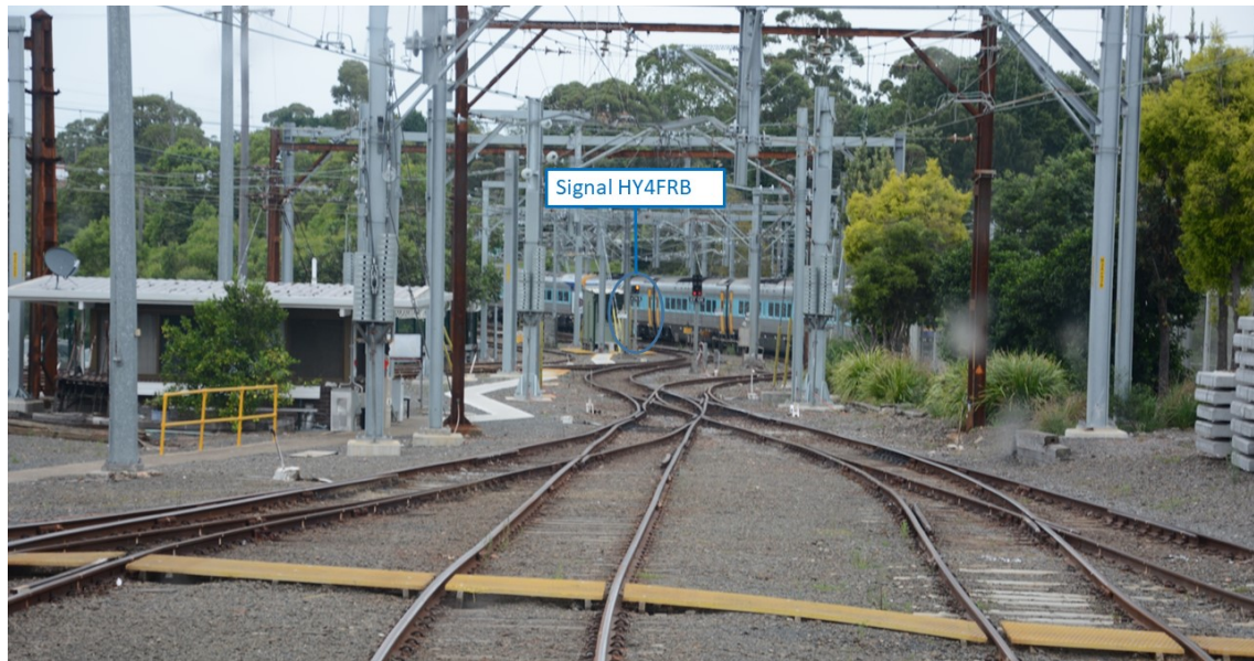
Figure 2: View from train driver’s cab to signal HY4FRB at HMC
