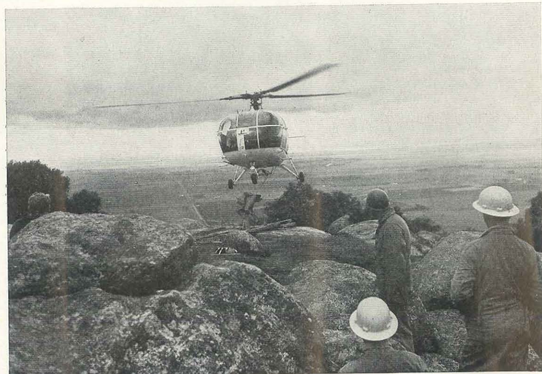
COVER AND ABOVE: Jayrow Helicopters' Sud Alouette unloads equipment at a rocky "helipad" in the You Yang Ranges, Victoria, during the construction of an aeronautical hazard beacon on Flinders Peak.
