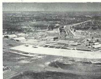
The New Passenger Terminal Loading Apron — Perth Airport.
