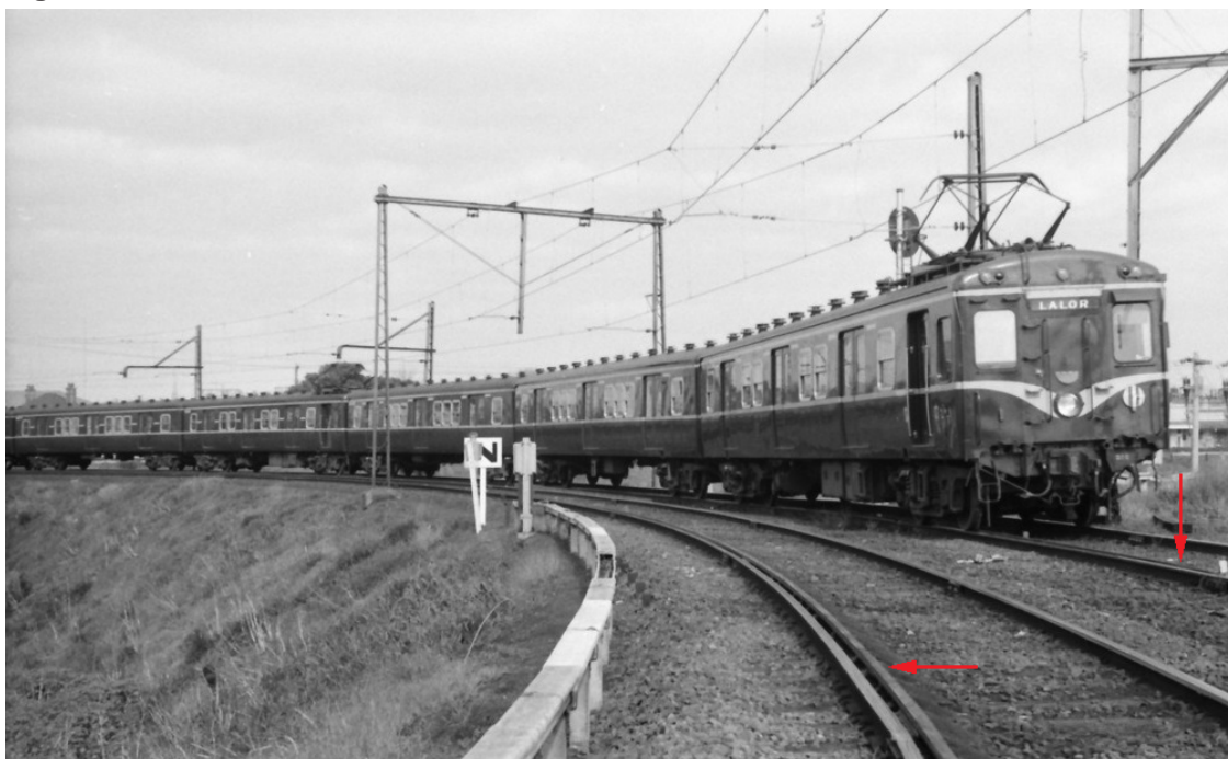
Figure 29: Historical use of check rails on Rushall curve c1965.
