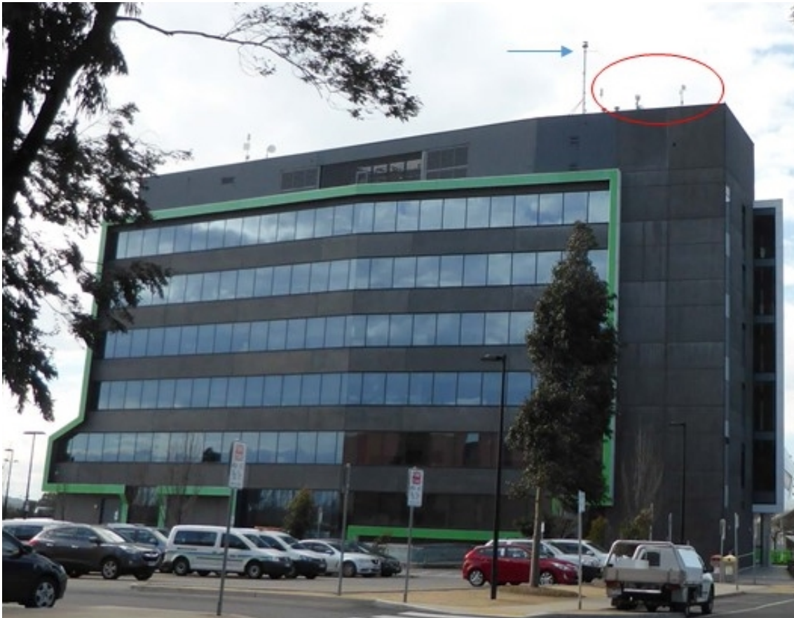
Figure 1: Hume City Council building showing the existing antennas (circled in red) and the (then) proposed radio mast (indicated with a blue arrow).
