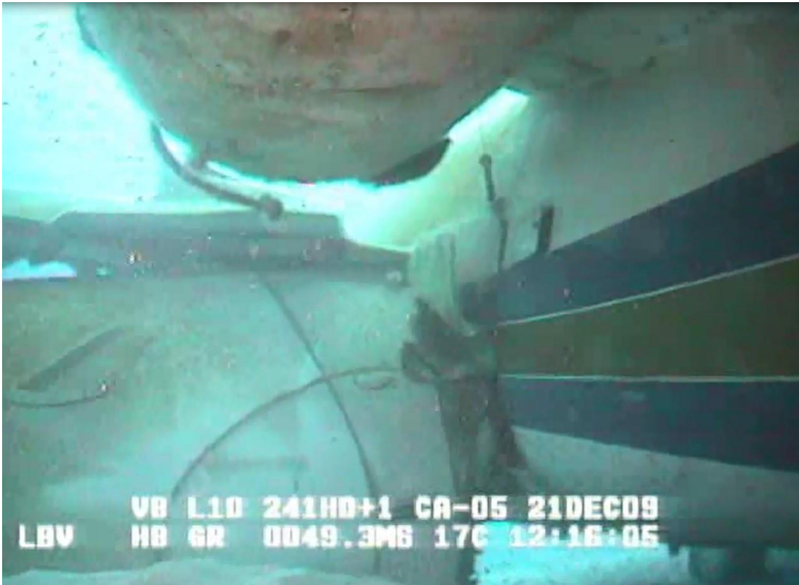
Figure 21: View looking forward from under left engine showing hydraulic damage to lower half of forward baggage compartment door.
