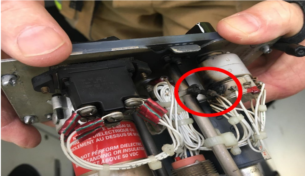
Figure 1: Burnt potentiometer in the aileron/rudder trim control panel (circled in red)
