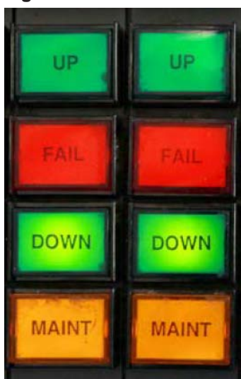
Figure 2: Tower control console hookcable pushbuttons
