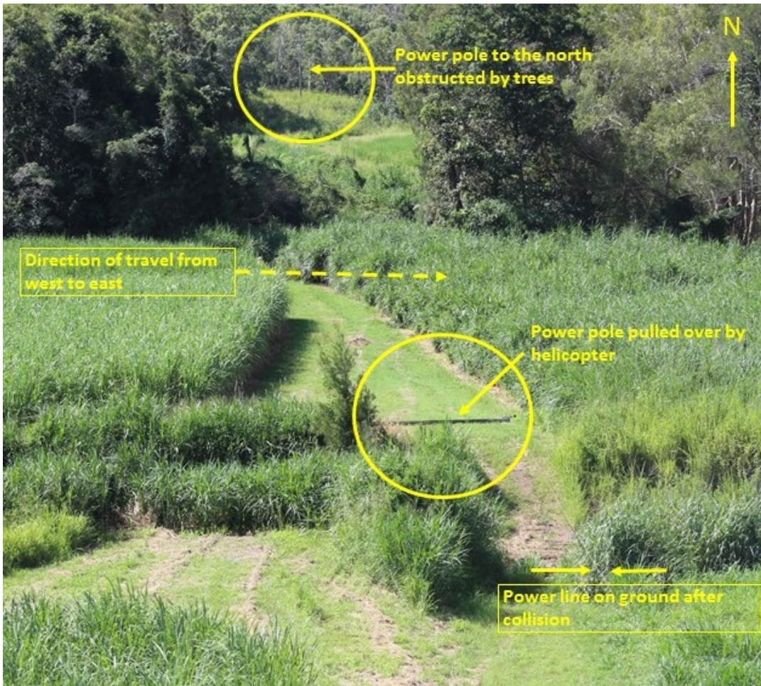
Figure 3: Terrain in the vicinity of the powerline, showing the helicopter’s direction of travel and the powerline and associated poles. Note the power pole that has been pulled down as a result of the wirestrike (centre of the picture) and the tree-lined creek that tracks right to left (located towards the top of the figure)
