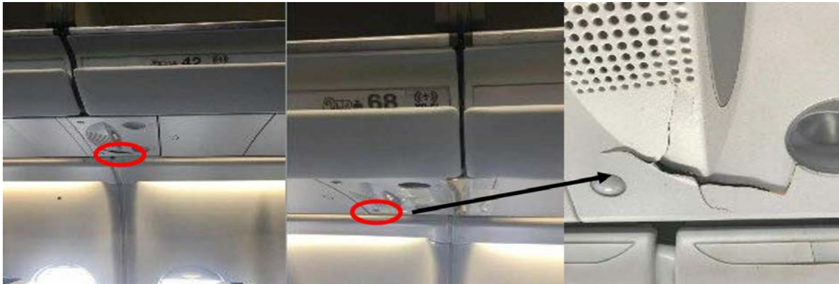
Figure 1: Damage to cabin (row 42, and 68 passenger service unit)
