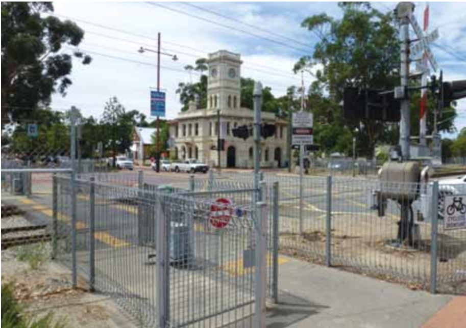
Figure 12: Meadow Street level crossing and pedestrian gate
