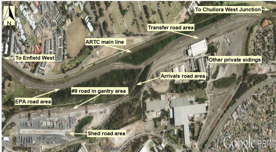
View of the Pacific National Sydney Freight Terminal showing the relative location of the EPA and Gantry road areas. The uncontrolled movement of locomotives NR24 and NR12 commenced at the #9 road in the gantry area before travelling through the transfer road area and toward Chullora West Junction. Source: Google, annotated by ATSB
