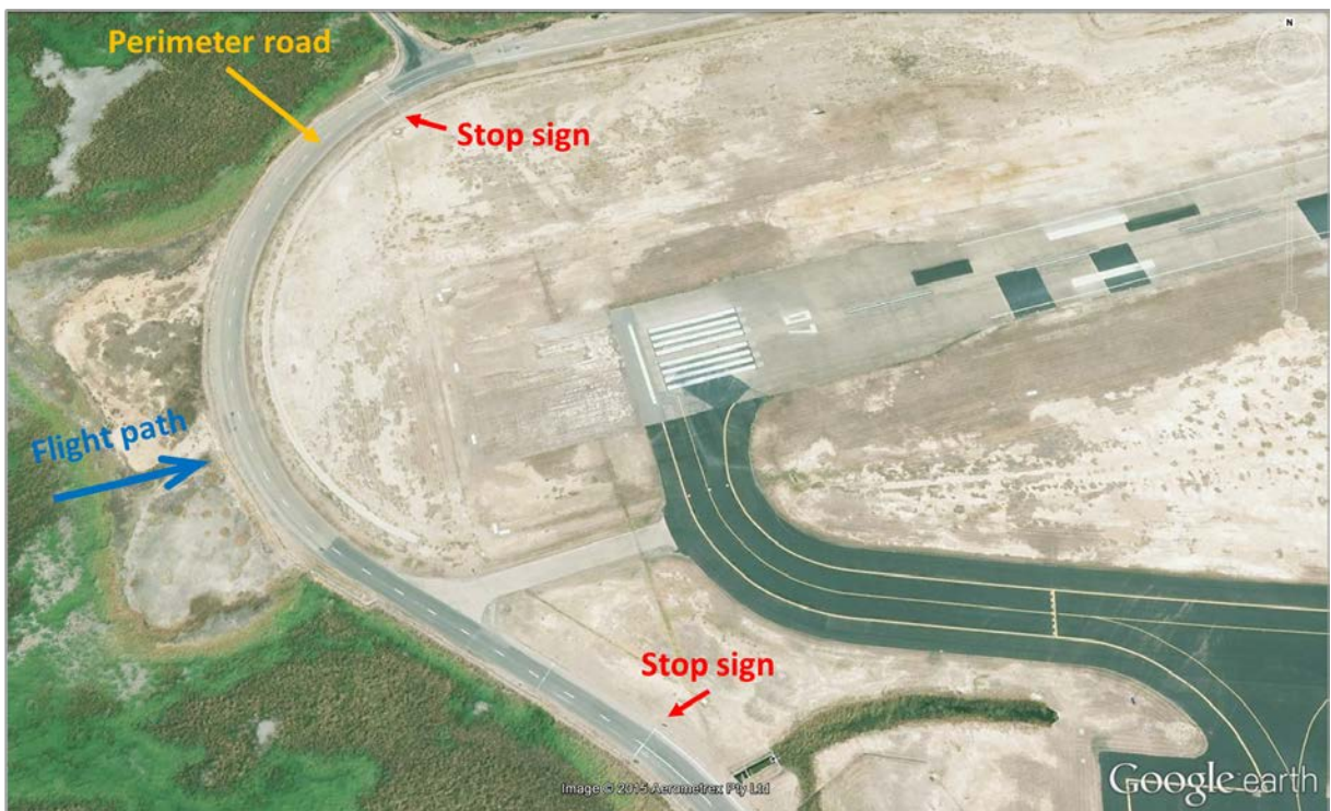
Figure 1: Townsville airport perimeter road near runway 07
