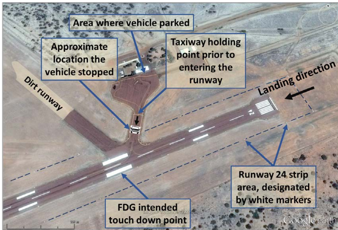
Figure 1: Blackall airport runway 24
