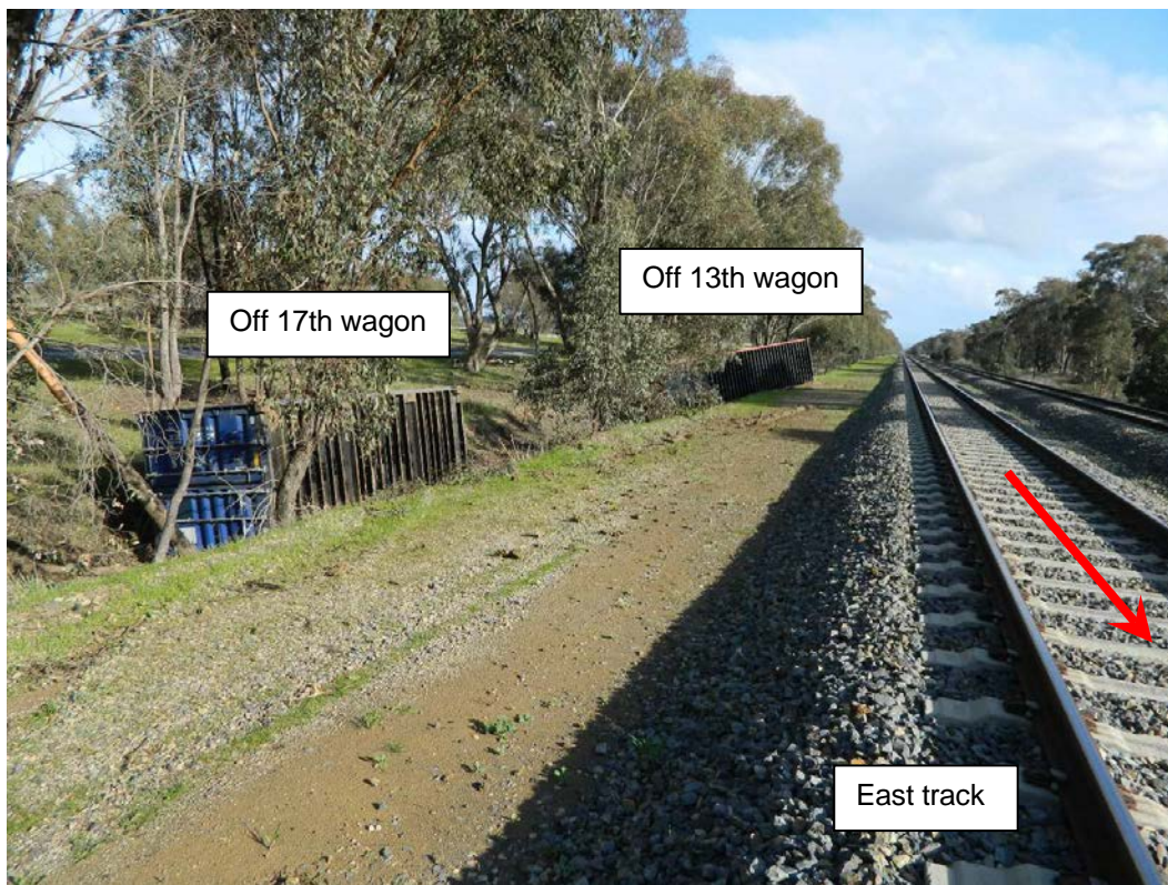
Figure 1: Containers laying adjacent the track
