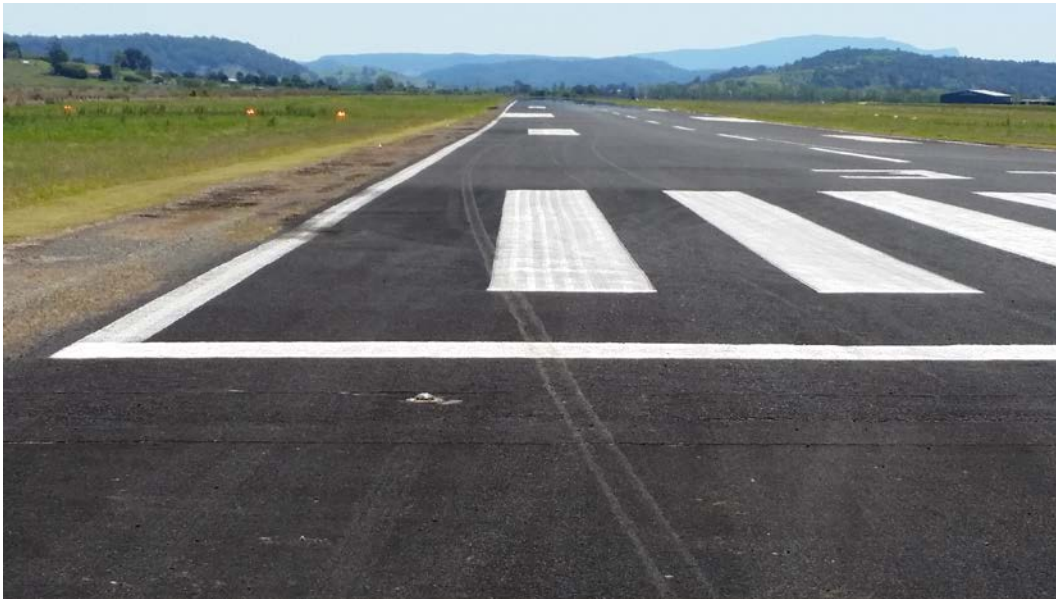
Figure 5: Southeast end of the runway showing right wheel contact marks on the runway and their position in relation to the runway centre line
