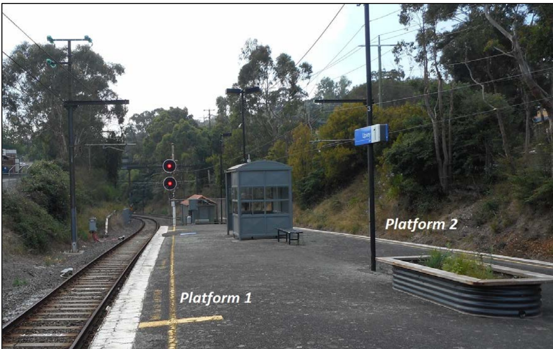
Figure 4: Upwey railway station looking towards Upper Ferntree Gully and signal No 42
