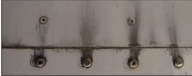
Figure 2: Typical indication of working rivets (photograph not of a CH-7B helicopter)
