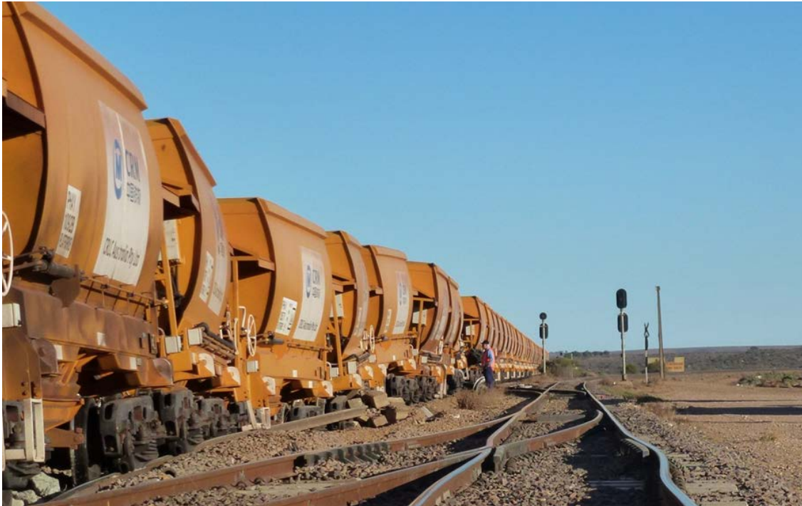
Figure 2: Derailment Inspection at Spencer Junction, Port Augusta, South Australia
