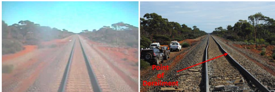
Figure 7: Video image from train 4414 (left) and photo post derailment (right)
