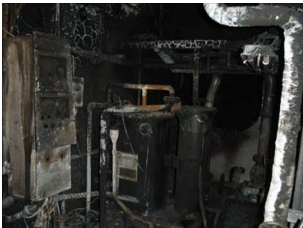
Figure 10: Oily water separator
