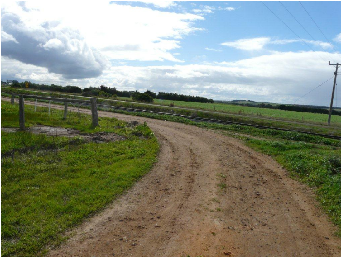
Figure 2: Intersection of Gallagher Road and the access track
