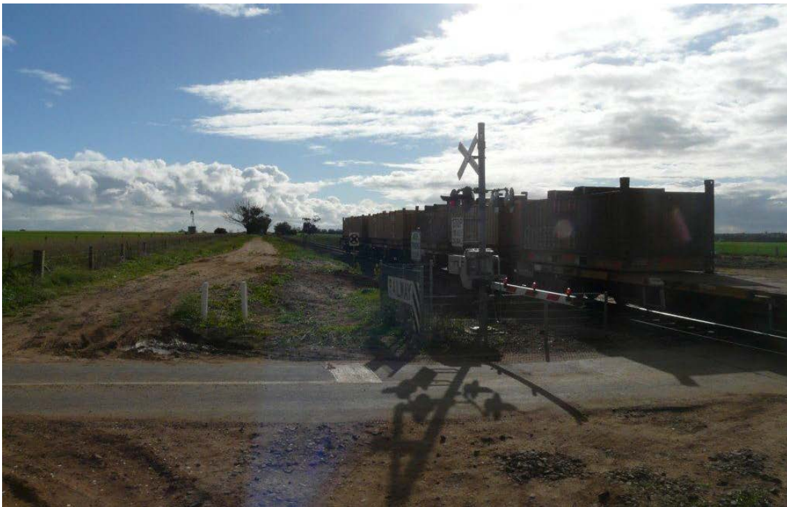
Figure 5: Approaching level crossing from access track
