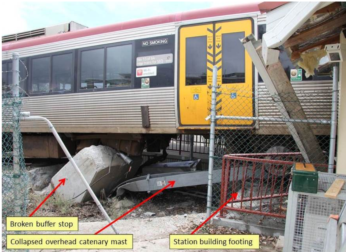
Figure 2: View of lead passenger car bridging the buffer stop and the overhead catenary mast.
