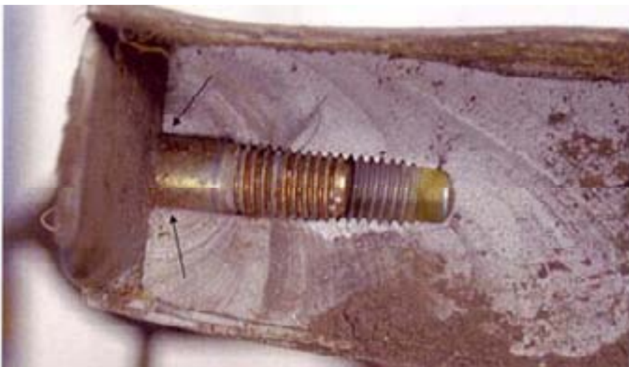
b) "The arrows indicate the location of the fracture origins on both sides of the bolt hole very close to the leading edge"
