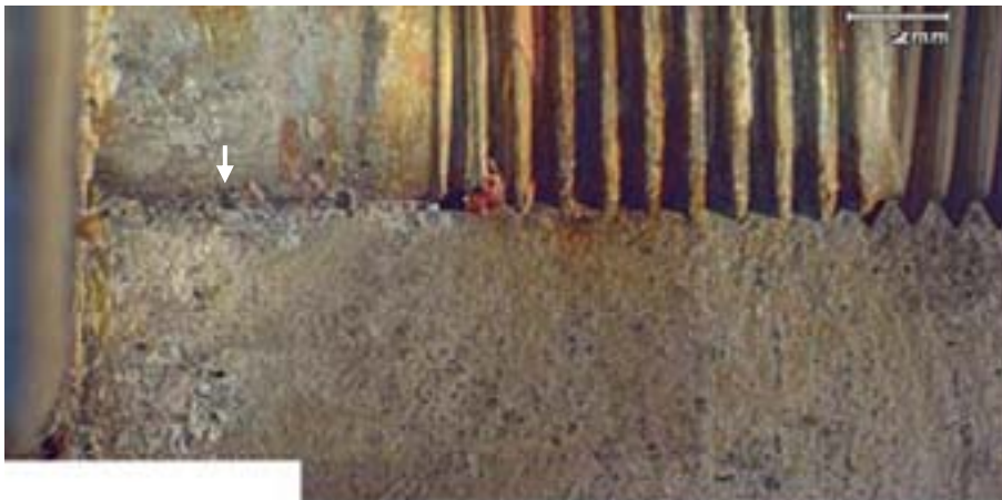
b) Lower side of the bolthole with the bolt in situ. The site of fatigue crack initiation is arrowed
