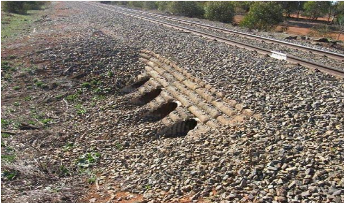
Figure 8: Roto Culvert, northern side view 12
