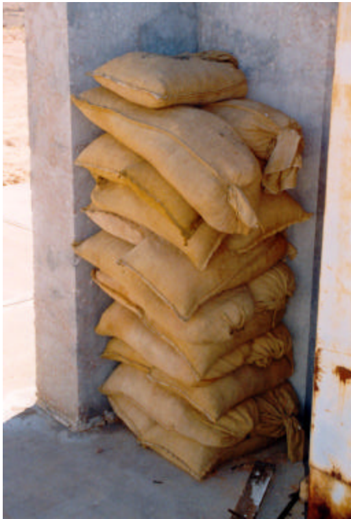
Fig. 57 (above). Sand bags typical of those used around the base of the launcher pedestal, in lieu of the grouting.
