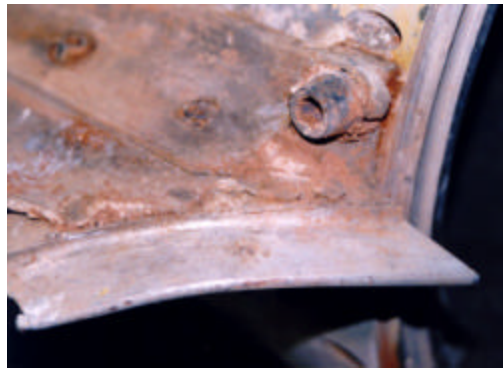
Fig. 24. Tip of the leading edge strip shown in figure 23. No evidence of thermal damage, although the skin behind is partially melted and eroded.
